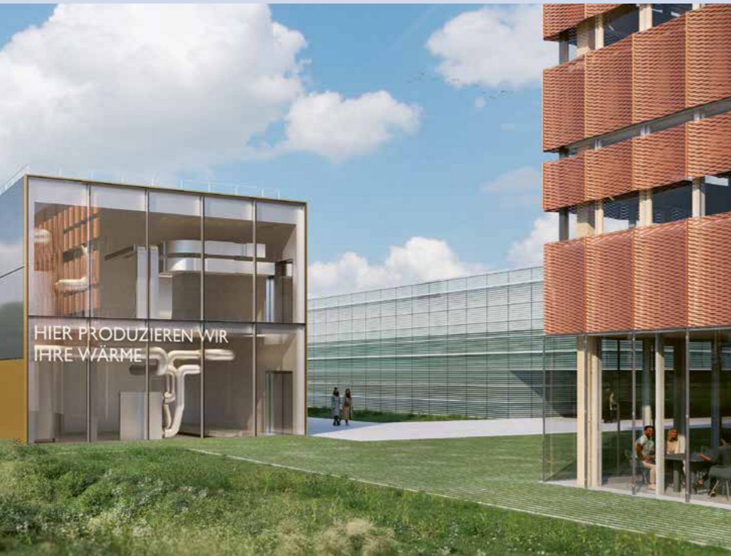
Construction has begun on HLRS III, a new data center in Stuttgart. The new facility will include a waste heat processing center, seen at the left of this rendering, which will capture all waste heat generated by the center's supercomputers and distribute it to the district heating network of the University of Stuttgart campus.
