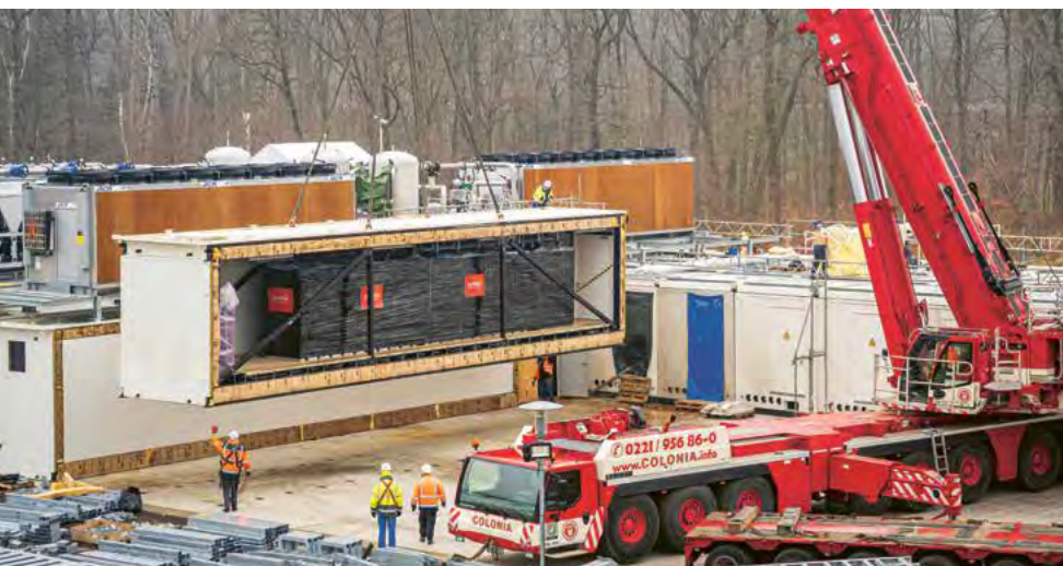
Delivery of an IT Module built of two containers, each container housing 10 racks.
