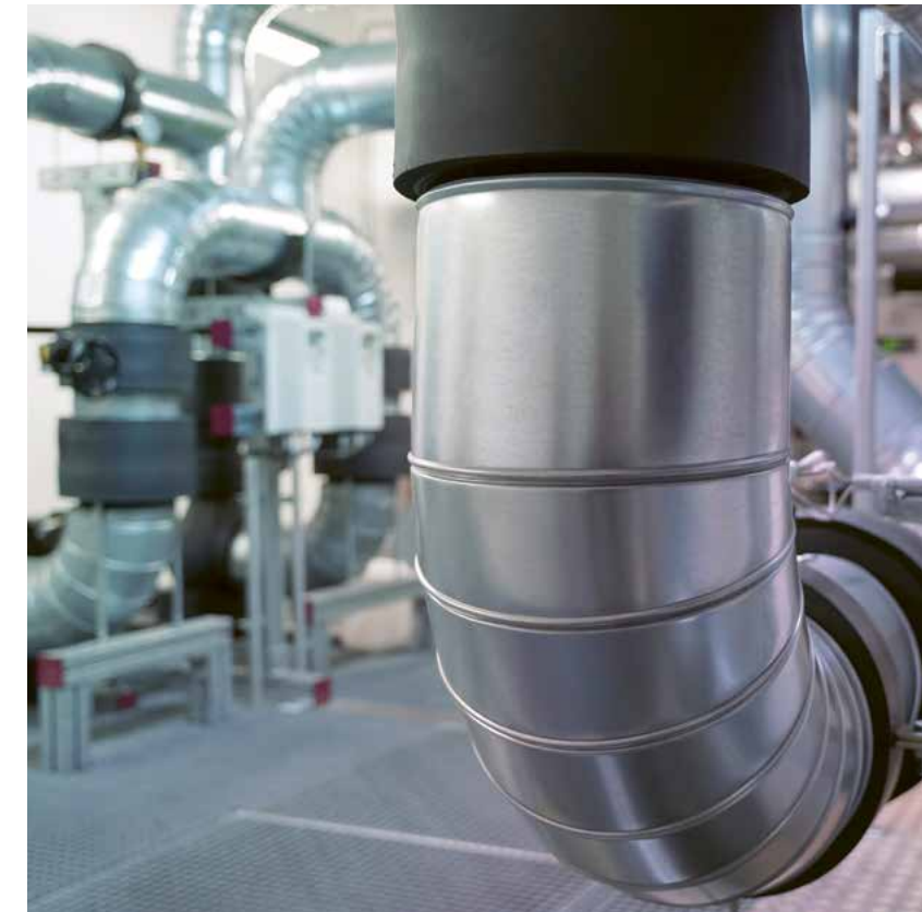
LRZ has long used warm-water cooling to improve the energy efficiency of operating its supercomputing systems. Its latest system, SuperMUC-NG Phase 2, the power supply units are also directly cooled with warm water, allowing the center to nearly create room-neutral system operation.
