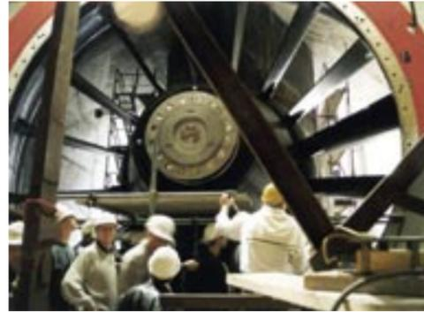
Figure 1: Wicket gate of bulb turbine in Ruppoldingen power station, generator housing in the background (Aare-Tessin AG, CH).  $\Delta$  6m, P=9.5 MW
