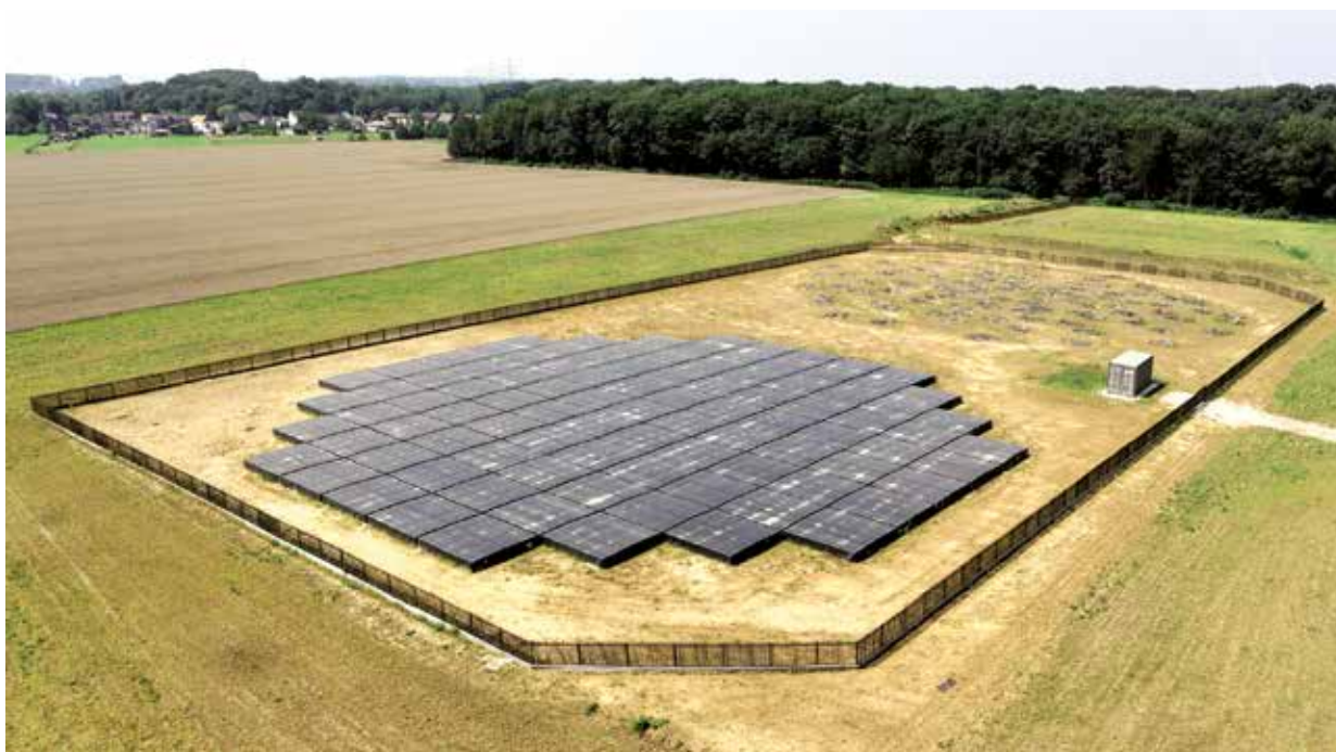
Jülich's LOFAR station DE605 consists of two antenna fields for measuring high and low frequencies. The container between them houses the electronics for processing the signals from the individual antennae.
